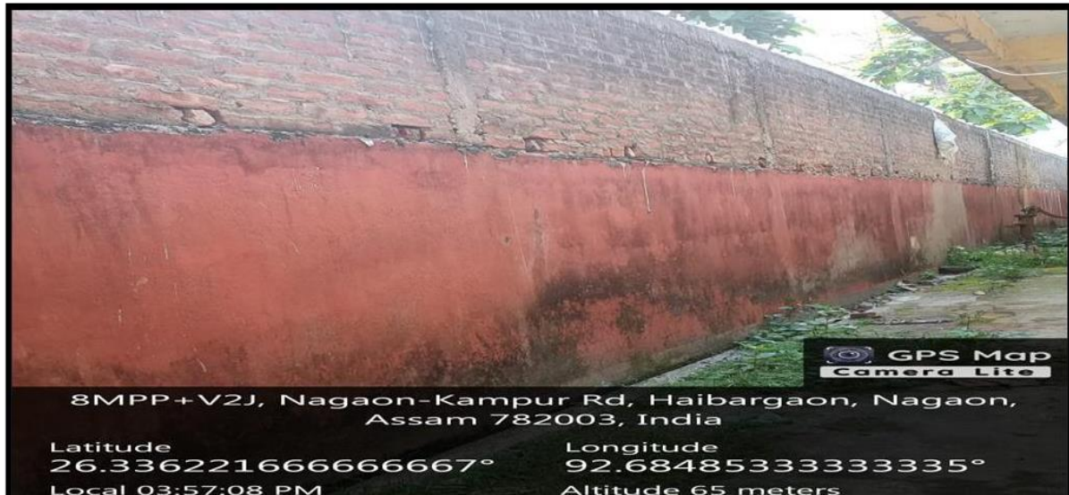
Figure 4. Fire Extinguisher and High Walls at the Girls' Hostel
