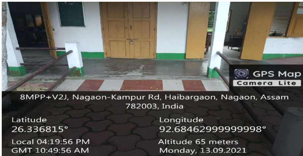
Figure 39. Ramps at different location on the campus
