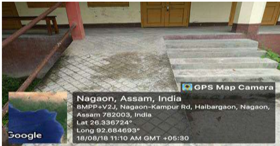
Figure 40. Photograph of Railing facility at the campus
