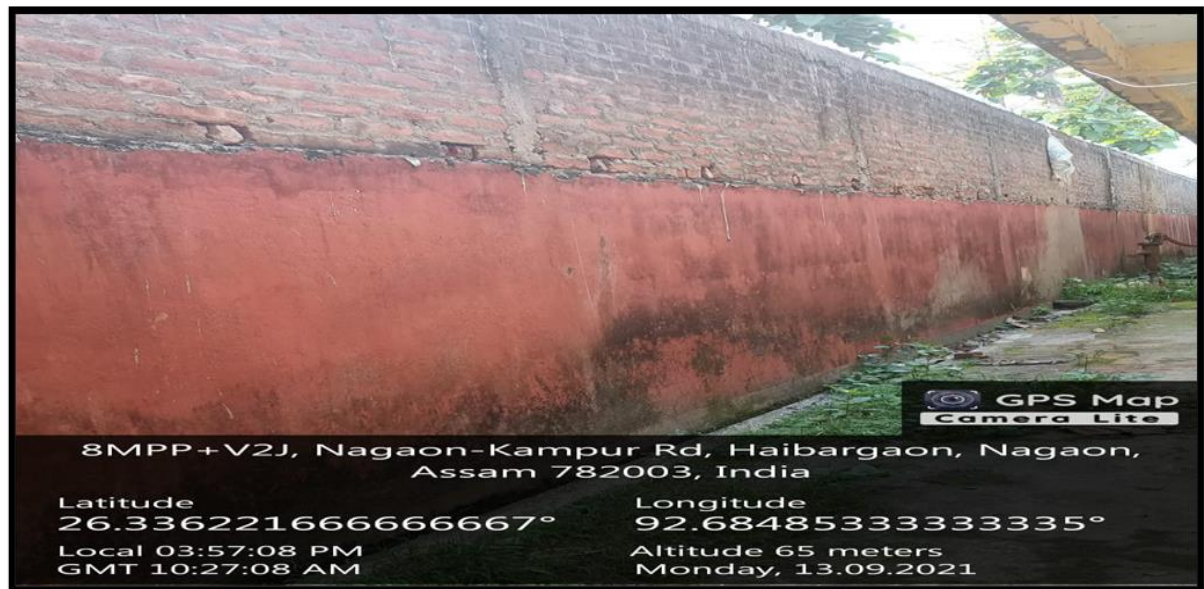
Figure 4. Fire Extinguisher and High Walls at the Girls' Hostel
