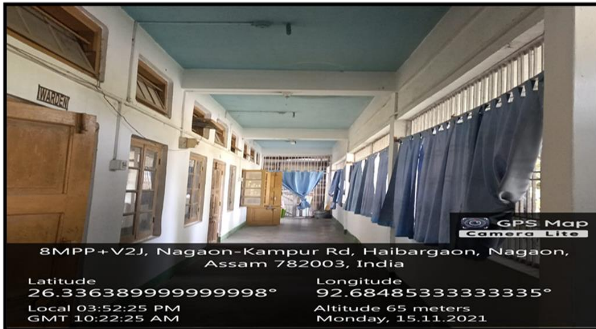
Figure 3. Girls' hostel corridor with iron grills
